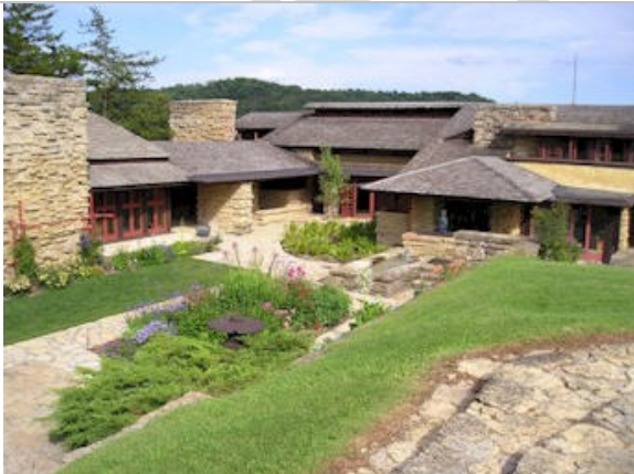
Prairie House Example - Taliesin's drafting studio by Frank Lloyd Wright. Picture by K. Murphy.
