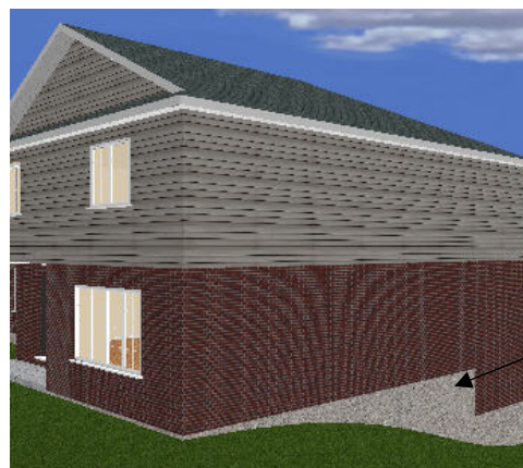
Daylight Basement with the foundation wall exposed.
